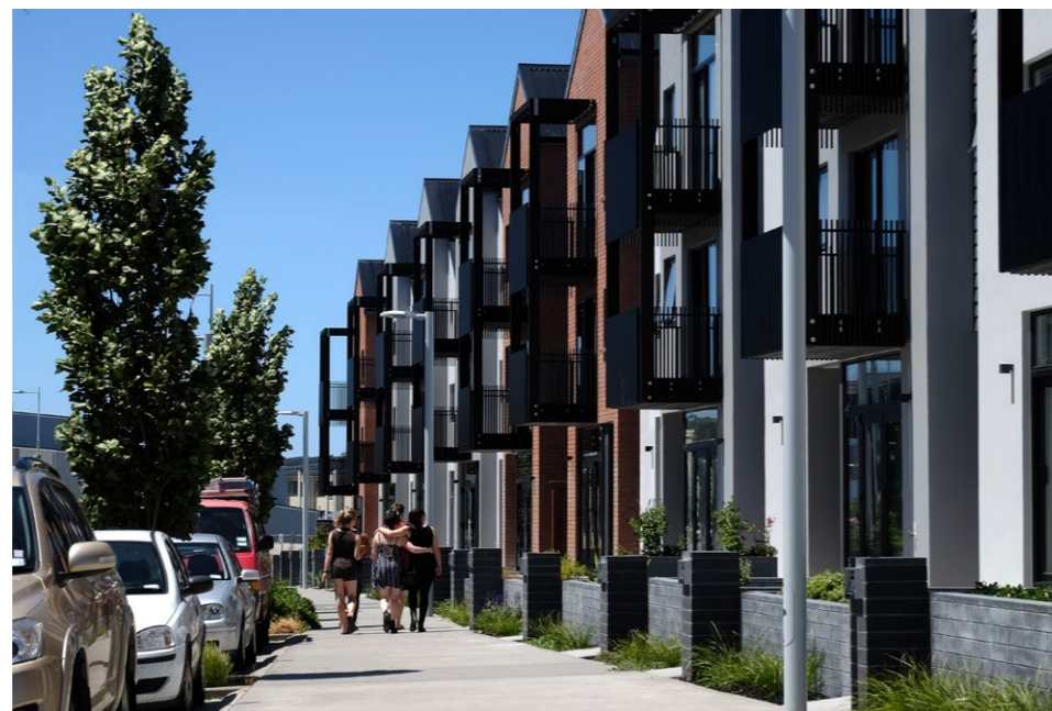
Image. Positive streetscape and building frontages.
