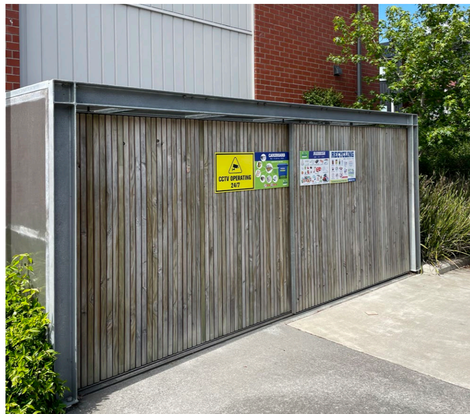
Above image. Hobsonville Point, Auckland. Communal bin store is conveniently located and well ventilated.
