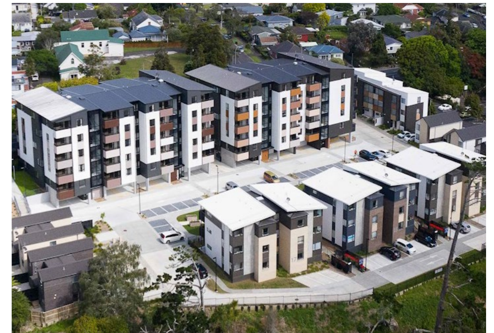
Above image. Undercroft parking as a response to slope. Note surveillance from open space and housing opposite.
