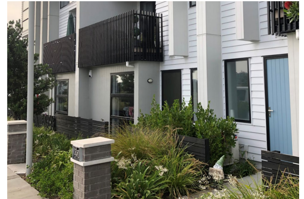
Above image. An upper-level balcony with northern aspect provides primary outdoor space that delivers privacy and connection to the street.
