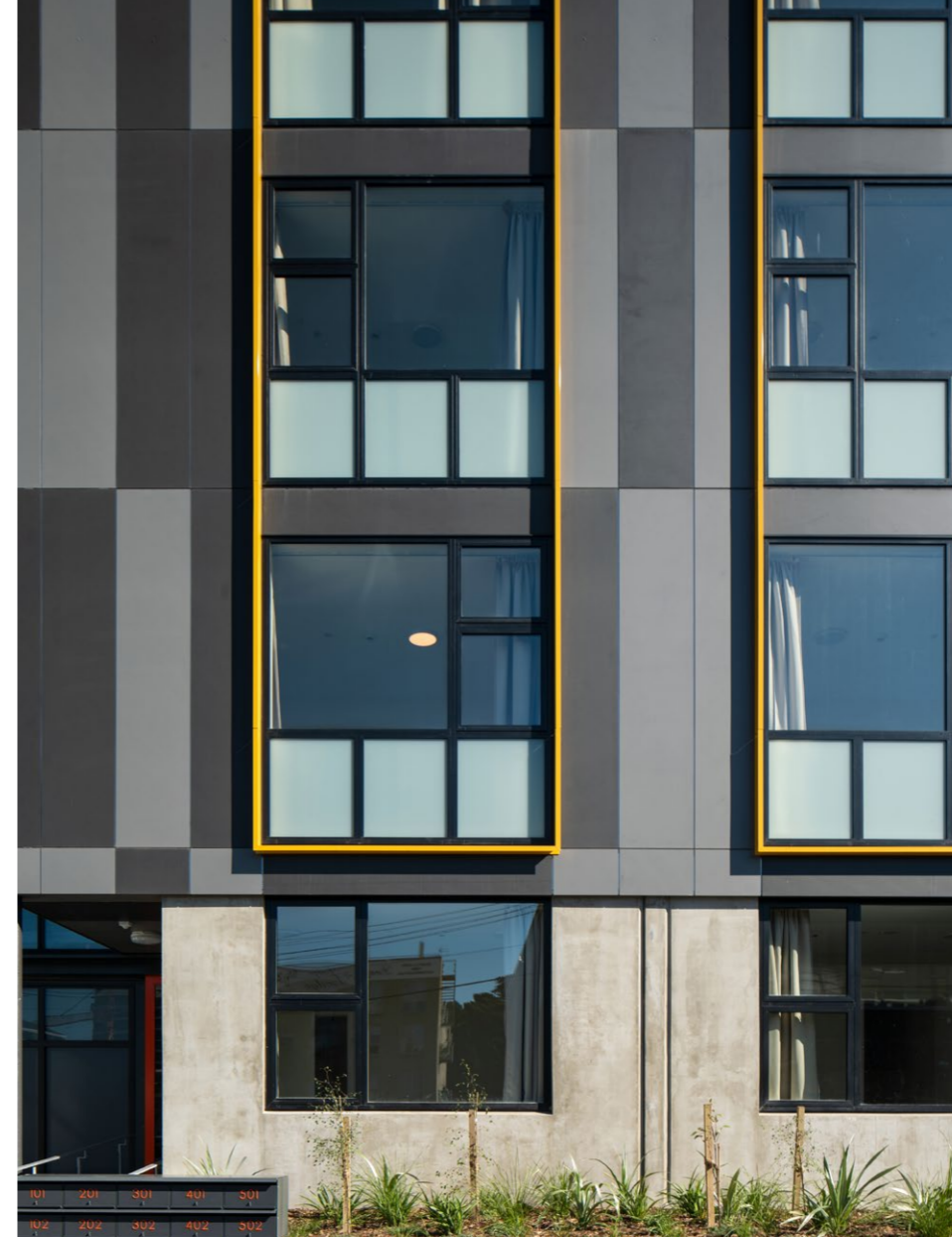
Left image. Good visibility over the street, bold façade design.
