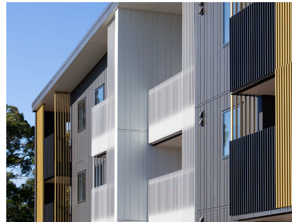
Left image. Recessed balconies in combinations with screening. Photograph: Ross Keane SGA Ltd.
