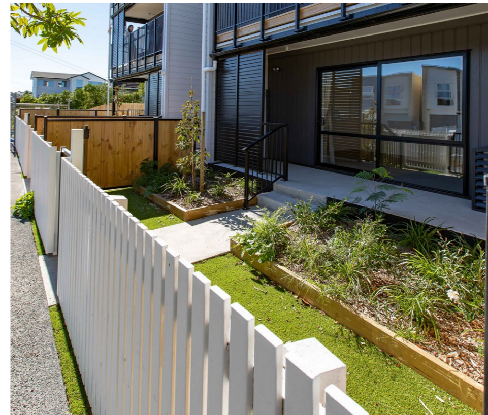
Left image. Where apartments front a street or open space, a gated connection can be provided for ease of access and greater activation of edges.
