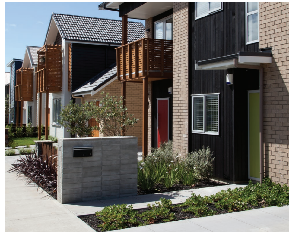
Left image. This south loaded terrace utilises ground-floor kitchen window and first-floor balcony to positively address the street.
