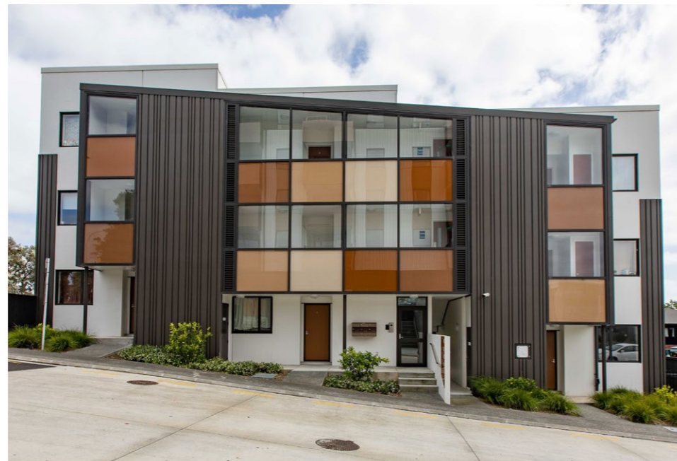
Image. Building slab is stepped down slope to ensure building entries are at, or just above road level. 1550 Great North Road, Waterview.
