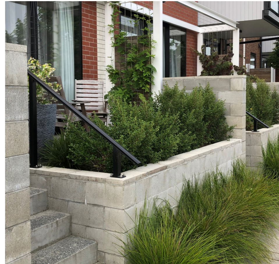
Left image. Well-used elevated private open space on the street front.
